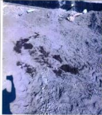
Spilled soil should be removed
