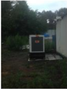
Running power generators outdoor without drip trays
