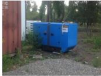
Running power generators outdoor without drip trays
