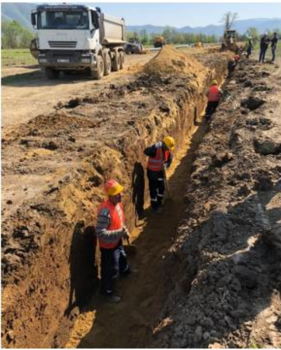
DN Pipe Laying – bedding layer preparation
