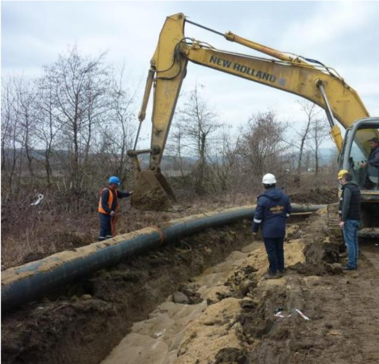
Construction of transmission main
