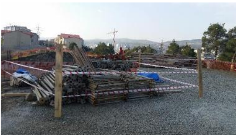
Office-01 – Storage of construction materials
