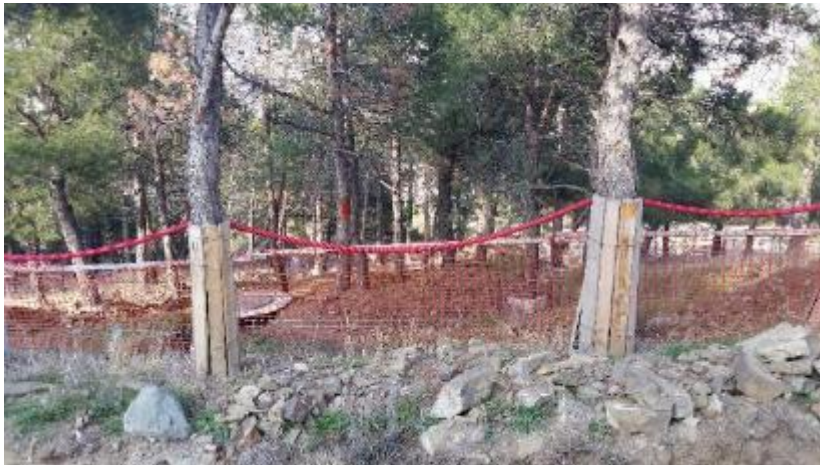
Office-01 protection of local tress
