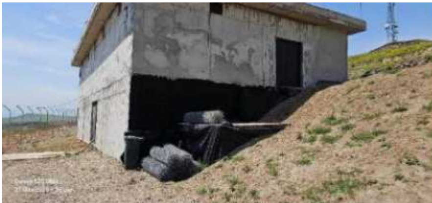
Photo N1 – City Reservoir
