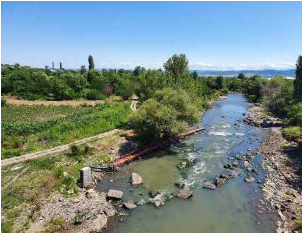
Photo N2: Damaged Sewerage Collector
