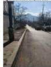
Fig.8: Removed Surplus Soil
