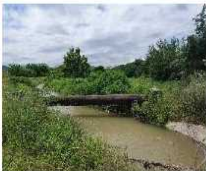
PS#1, WW Collector Photo No. 5
