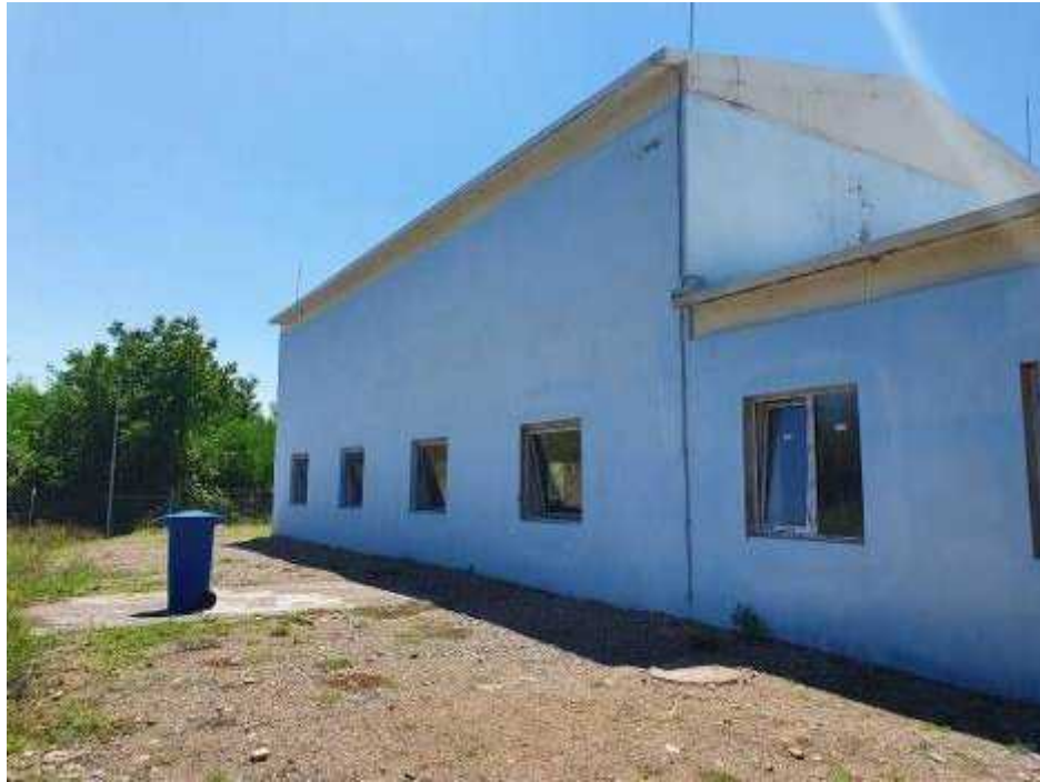
Photo N3 – MAR-01, LOT-06 Construction of Colagery wellfileds
