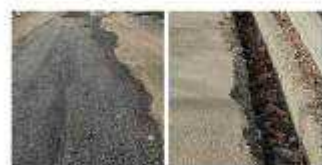
Fig.5: Roads during construction of Waste Water Network
