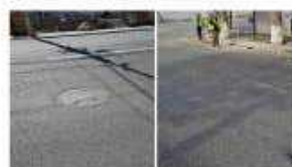
Fig.6: Roads after completion of construction Works
