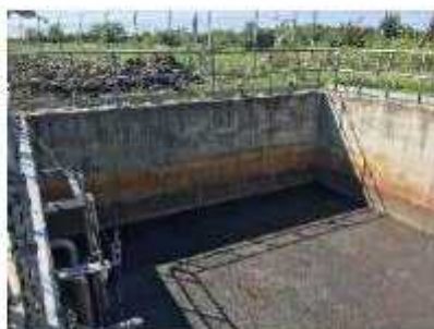
Drainage pump sum with scum layer after excavation end September 2023
