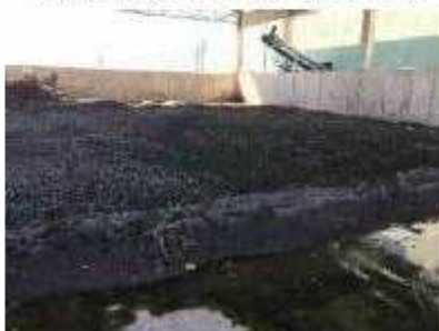
Sludge storage area
