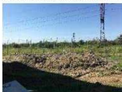
Sludge dump next to storage hall
