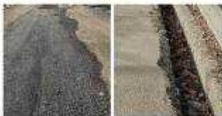
Fig.5: Roads during construction of Waste Water Network
