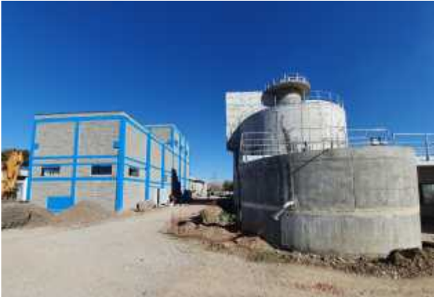
Photo N3, Marneuli WWTP
