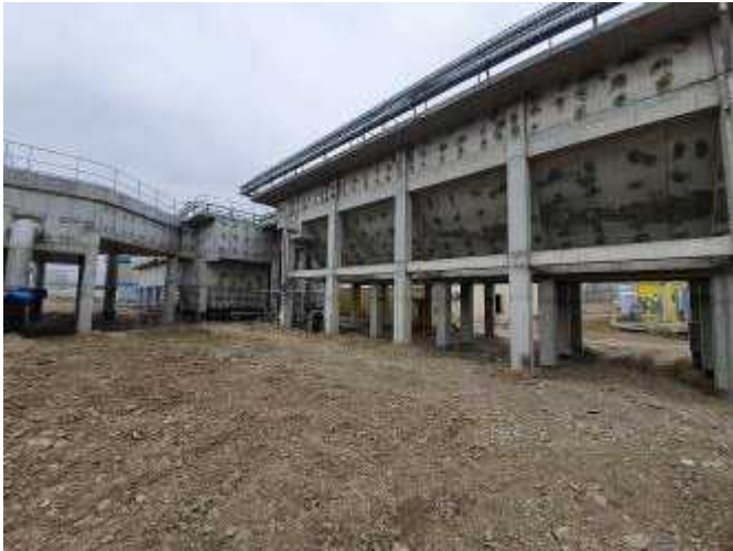
Photo N1 Marneuli WWTP
