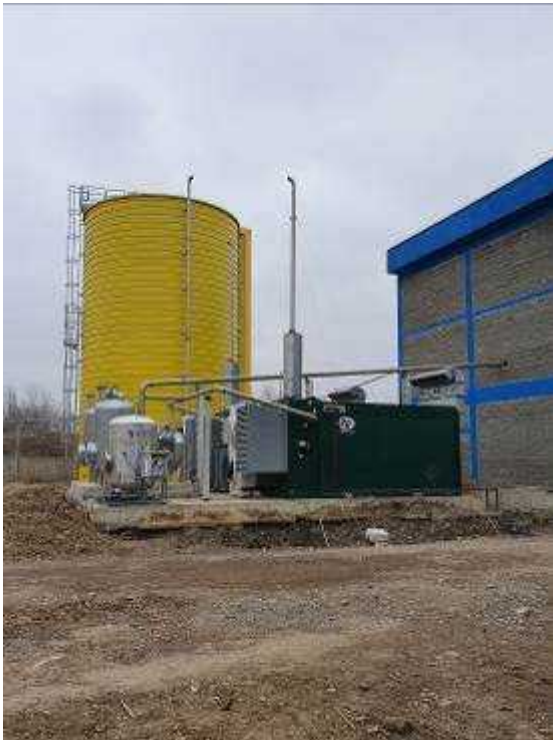
Photo N2 Marneuli WWTP
