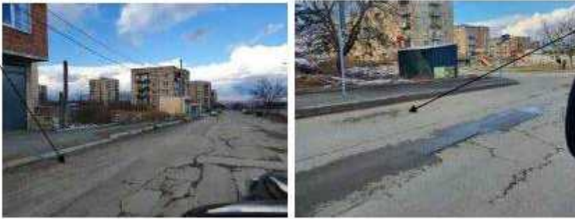
Water Supply Network Reinstatement Area (Fig.12,13)
