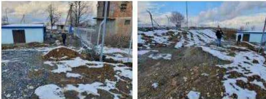
Vardisubani Pumping Station (Fig. 10,11)
