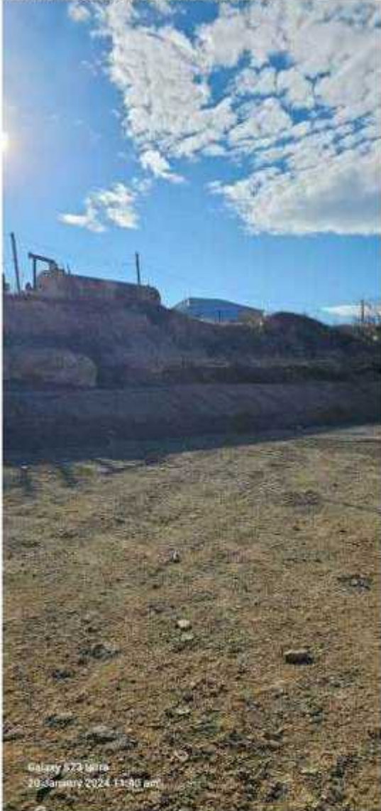
The part of fence are removed.
