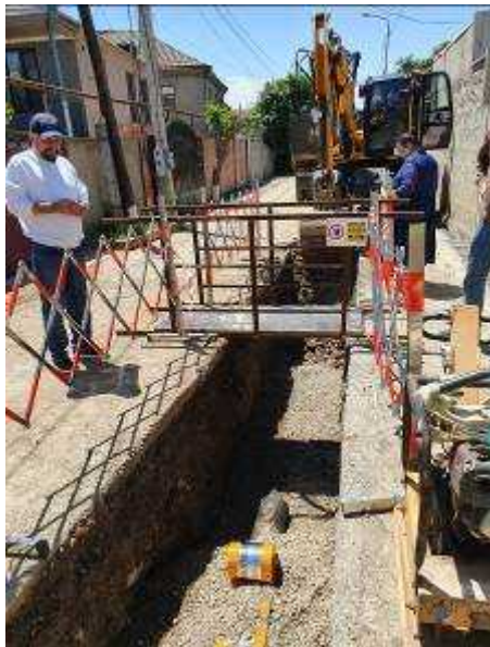
Photo N3 – Construction of the Sewerage Network
