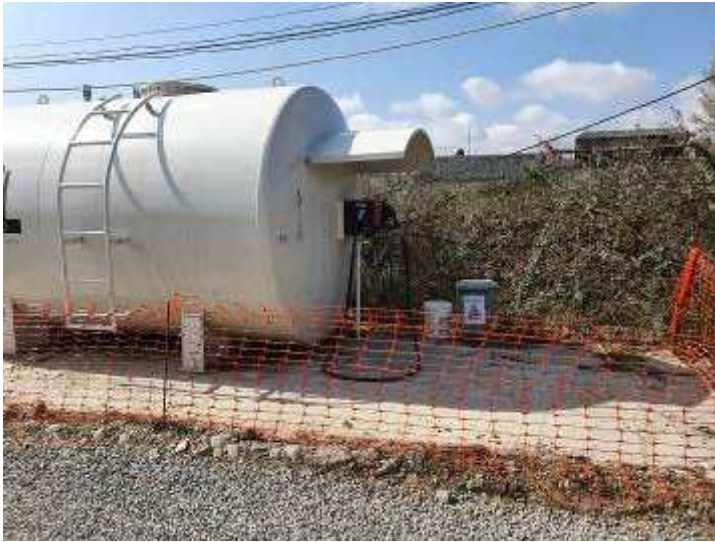
PHOTO N2 – MAR-01 – (LOT-01, LOT-02, LOT-03 and LOT-06), CAMP Site
