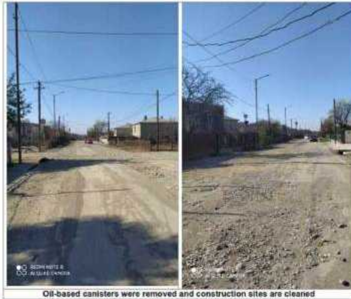
Oil-based canisters were removed and construction sites are cleaned
