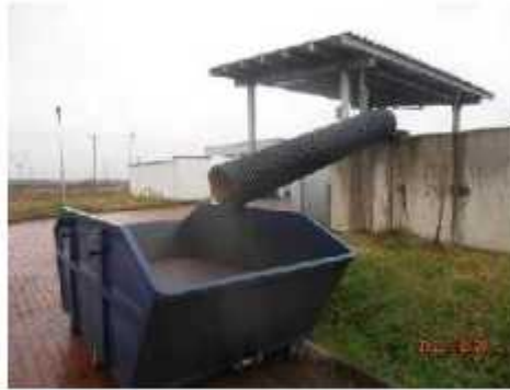
Dried sludge at emergency storage hall
