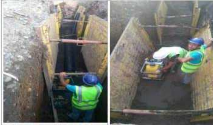
Walls of the deep trenches
