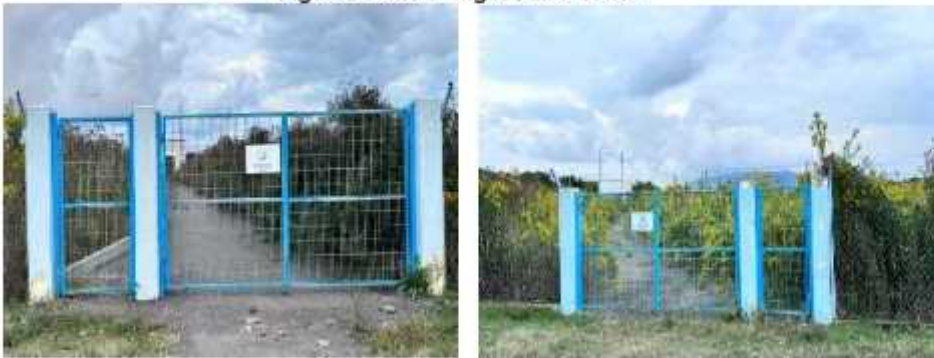
Figures 7 and 8: Ingiri Water Wells
