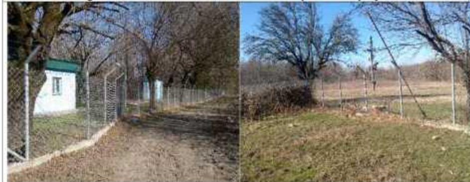
Figures 13 and 14: Area of wells fenced as part of the project
