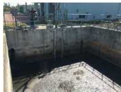
Drainage pump sump with scum layer after excavation end September 2023
