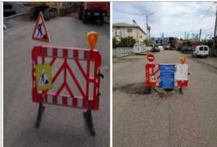
Construction activities signs
