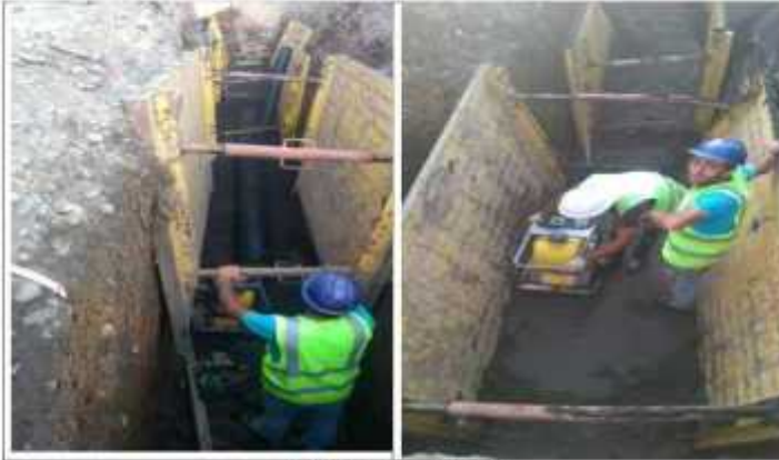
Walls of the deep trenches
