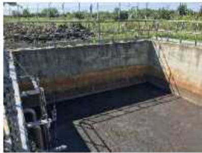
Drainage pump sump with scum layer after excavation end September 2023
