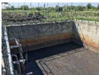
Drainage pump sum with scum layer after excavation end September 2023
