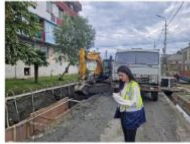
Figure 3.1 Noise (NM61) Monitoring Point
