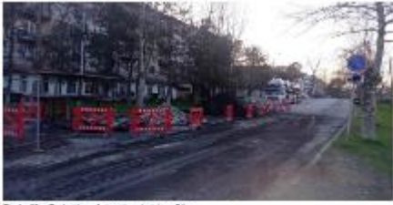
Photo #3 – Protection of stored material on 5th
