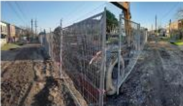
Photo #1 and Photo #2 – Site fence to protect the trenches installed
