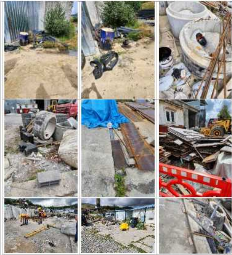
Temporary Storage Facility for Hazardous Waste
