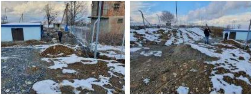
Vardisubani Pumping Station (Fig. 10,11)
