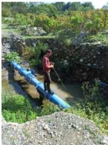
Worker without PPE/falling hazard
