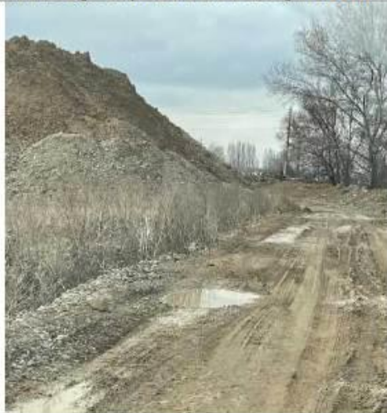
Photo 2: Muddy road and excavated materials
