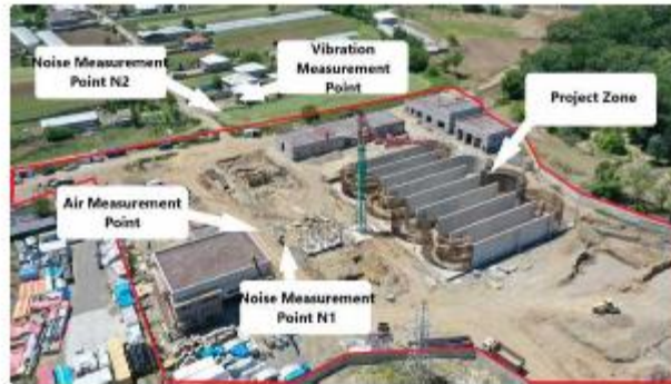
Construction of a waste water treatment plant in Marneuli
