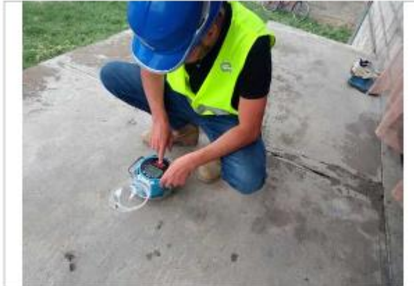
Construction of a waste water treatment plant in Marneuli
