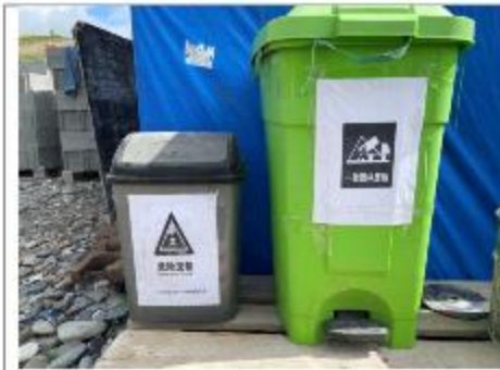
Hazardous and non-hazardous waste containers be installed at the site with proper labelling in Georgian and English language
