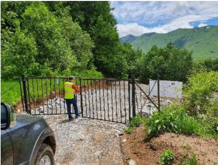
Construction of Gudauri Waste Water Treatment Plant N4
