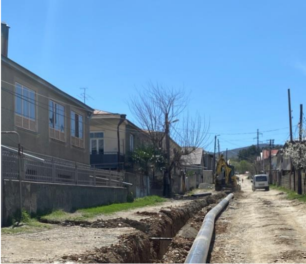
Excavation of pipeline trenches
