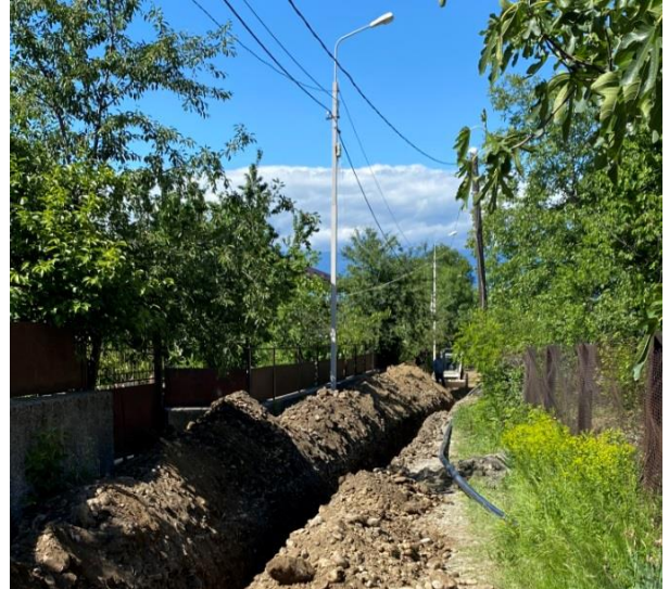
Excavation of pipeline trenches
