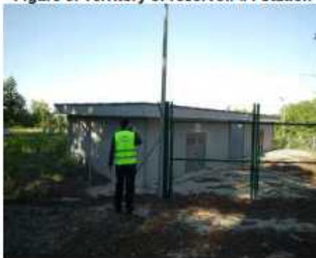
Figure 3: Territory of reservoir #1 station
