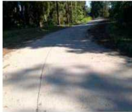
Figure 13: Access road to the pumping station
