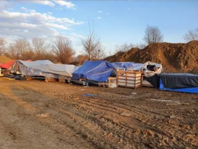
Construction and Rehabilitation of the Water Supply System in Chiatura (CHI-02)
