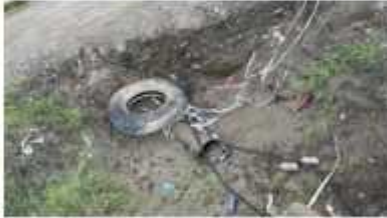
Open trench without hard barrier and warning signs
