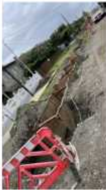
Open trench without hard barrier and warning signs
