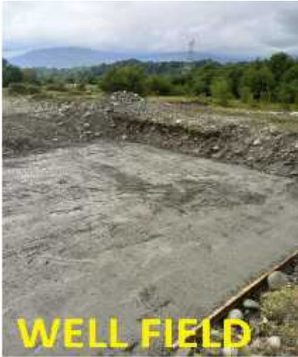
Construction of Well Field in Jvari, JVA-01, Photo N3
