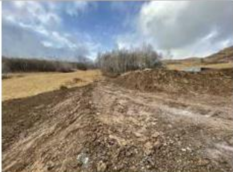
Site internally should be better arranged(better arrange on site internally)
