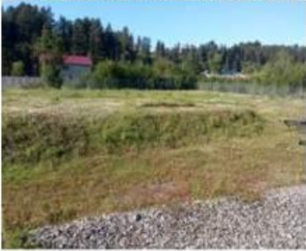
Figure 4: Territory of the pumping station
