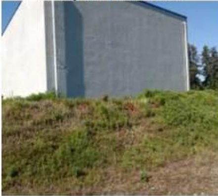
Figure 10: Self-restored grass – the territory of the first reservoir
