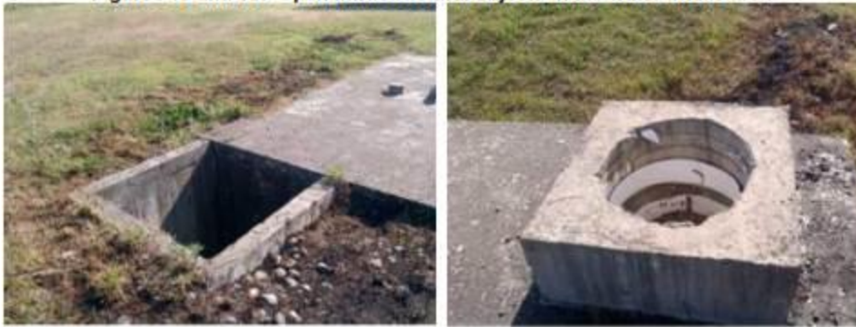
Figures 18 and 19: Open infrastructural objects in the water intake area
