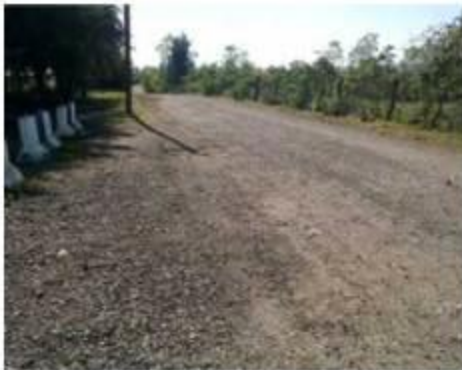
Figure 12: Access road to the first reservoir
