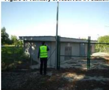
Figure 3: Territory of reservoir #1 station
