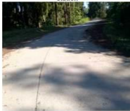
Figure 13: Access road to the pumping station
