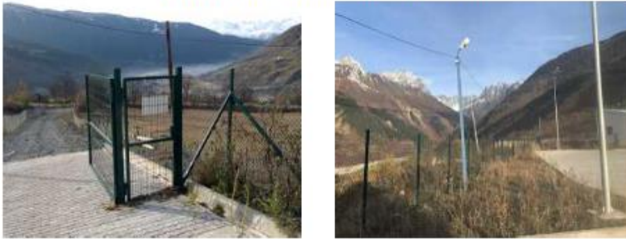
Figures 1 and 2: All project areas are fenced
