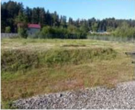
Figure 4: Territory of the pumping station
