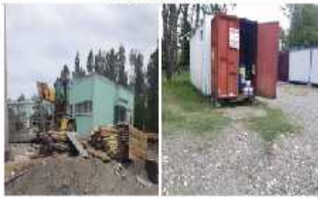
Figure 2: Construction site showing the foundation and early structure of the building.
