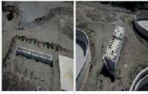
Figure 1: Construction site showing the foundation and early structure of the building.
