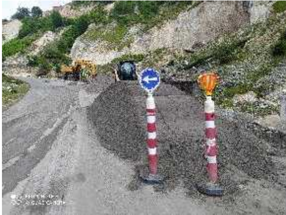
Construction of Water Reservoir in Jvari (Photo No5 Photo No6)
