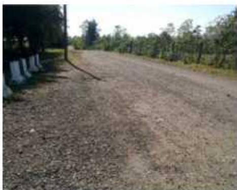
Figure 12: Access road to the first reservoir
