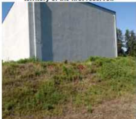
Figure 10: Self-restored grass – the territory of the first reservoir
