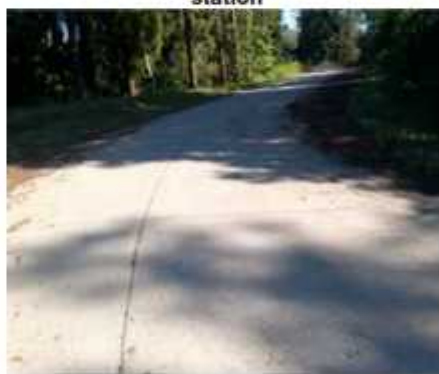
Figure 13: Access road to the pumping station
