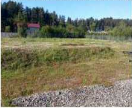
Figure 4: Territory of the pumping station
