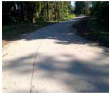
Figure 13: Access road to the pumping station
