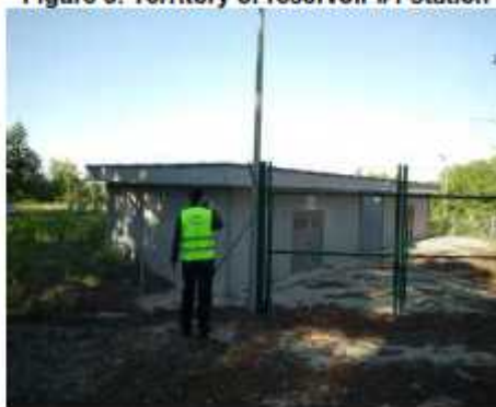
Figure 3: Territory of reservoir #1 station
