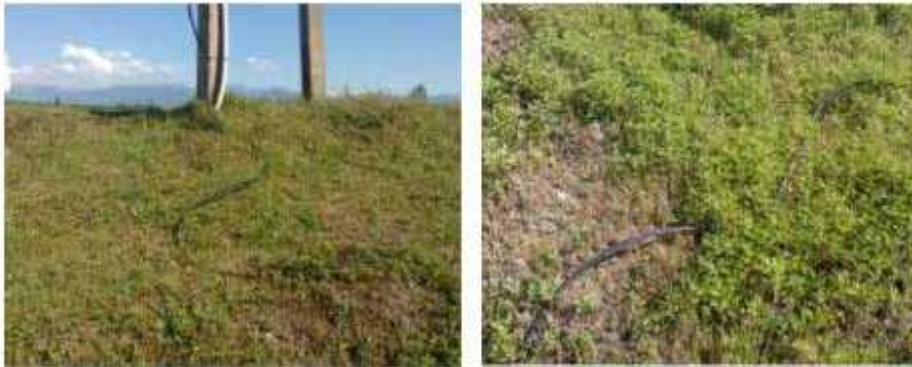
Figures 20 and 21: The wire cable on the earth surface
