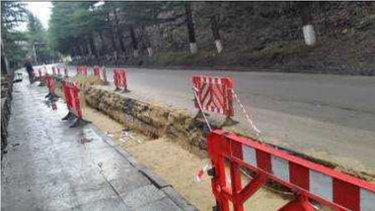
CHI-01 - Laying water supply pipes (Photo-02)
