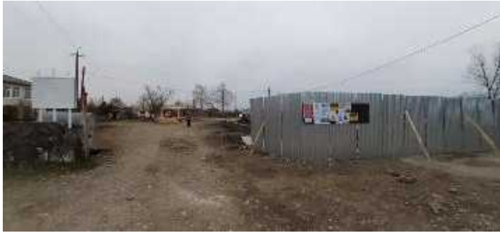
Abasha - UWSCG's Service Center area during construction; front view, Photo-01
