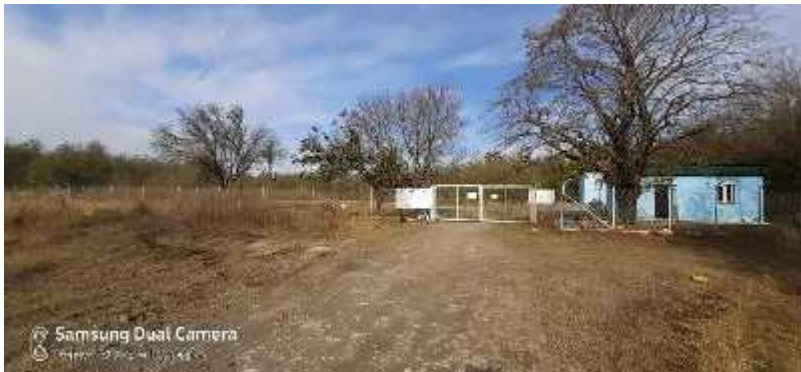
Abasha – Headwork, Rehabilitation of existing buildings for Well Field, Photo-03
