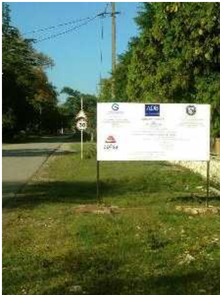
Abasha – City Distribution Network, Photo-02
