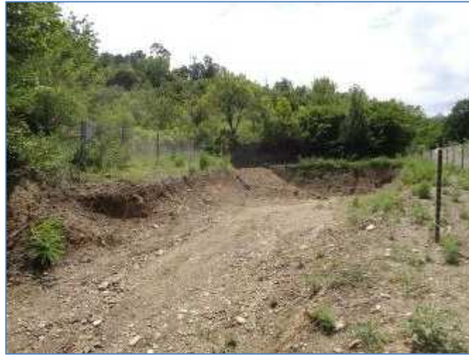
Figure 14: Photo of Borehole 7
