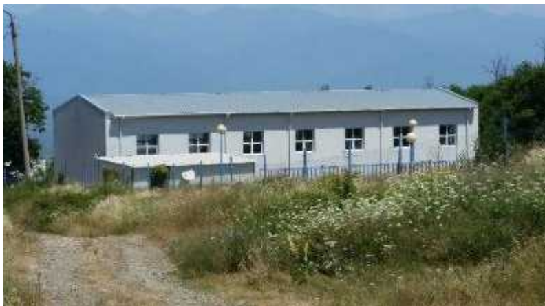
Photo of 1000m3 Reservoir on the University Street
