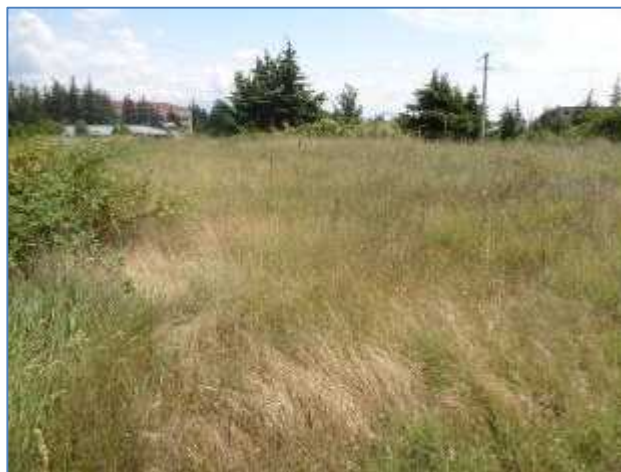
Figure 9: Photo of No2 – Reservoir with capacity of 2000 m 3
