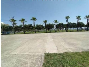
Figures 9: Restored asphalt layer near the "Anaklia" Hotel
