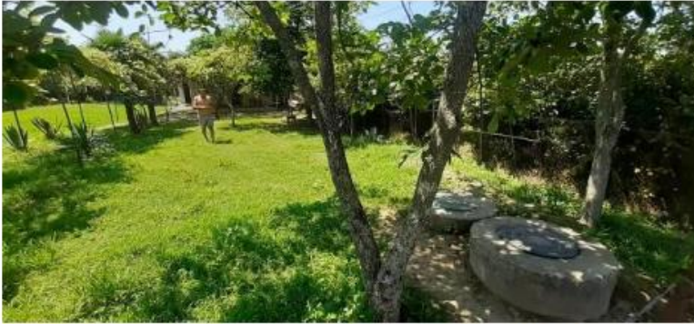
Connection of residential houses in Anaklia resort to main sewer line. Corrugated d=150mm
