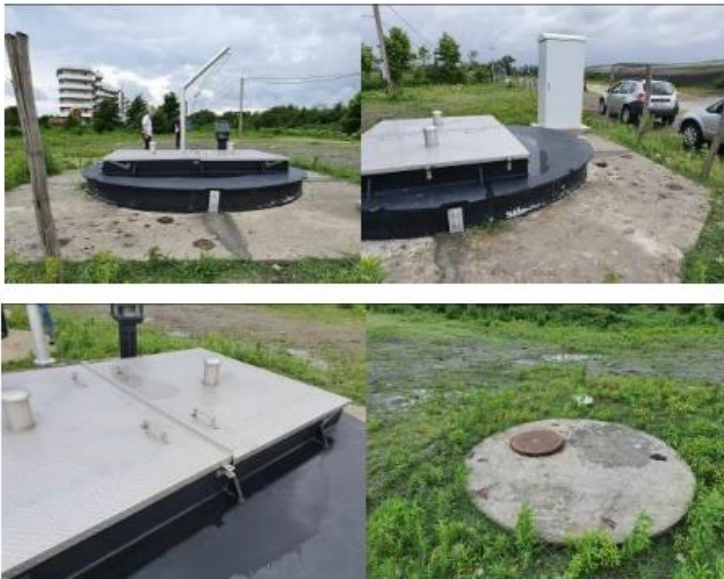
Figures 2: Reinstatement activities, Anaklia – Installed # 33 Pumping Stations (PS # 33);
