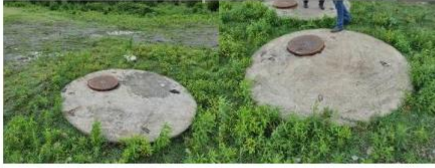
Figure 8. Underground Manholes in the vicinity of the PS N33
