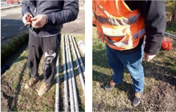
Worker without PPE at the construction site
