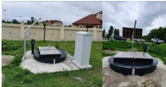
Figures 1: Reinstatement activities, Ganmukhuri – Installed # 22 Pumping Stations (PS # 22).
