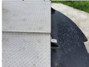
Figure 6. Pumping Station N22
