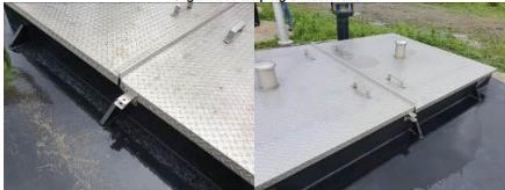
Figure 7. Pumping Station N33
