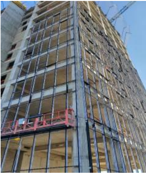
Photo: UWSCG Office Building, TBI-01
