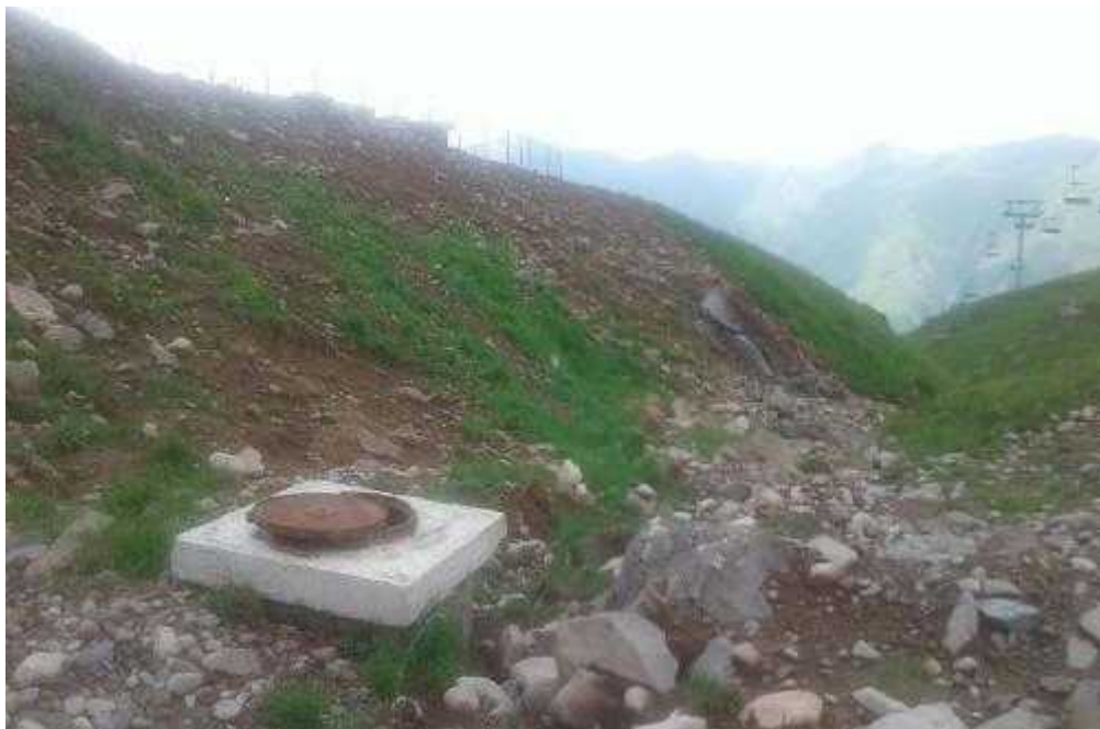
Figure 1. Existing Reservoir of Gudauri
