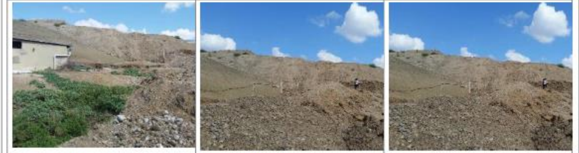
Photos of refilling of treches and diesel generator on site
