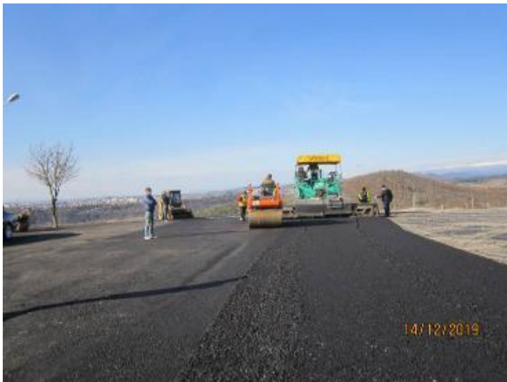
KUT-01 First layer of asphalt front of Godogani reservoir
