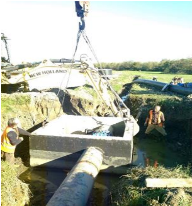
Photo: ABA-01 Construction of Network
