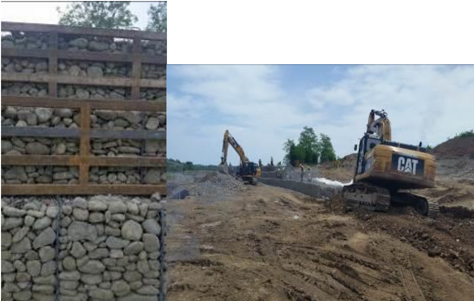
River Natanebi Gabion Protection Wall
