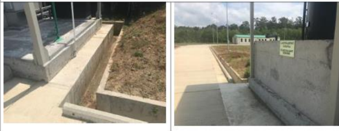
Figure 3 and 4: Drainage system in the project area
