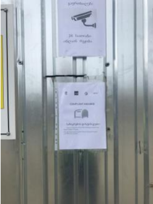
Photo: Construction of the Water Supply Network in Ureki (Ure-01)
