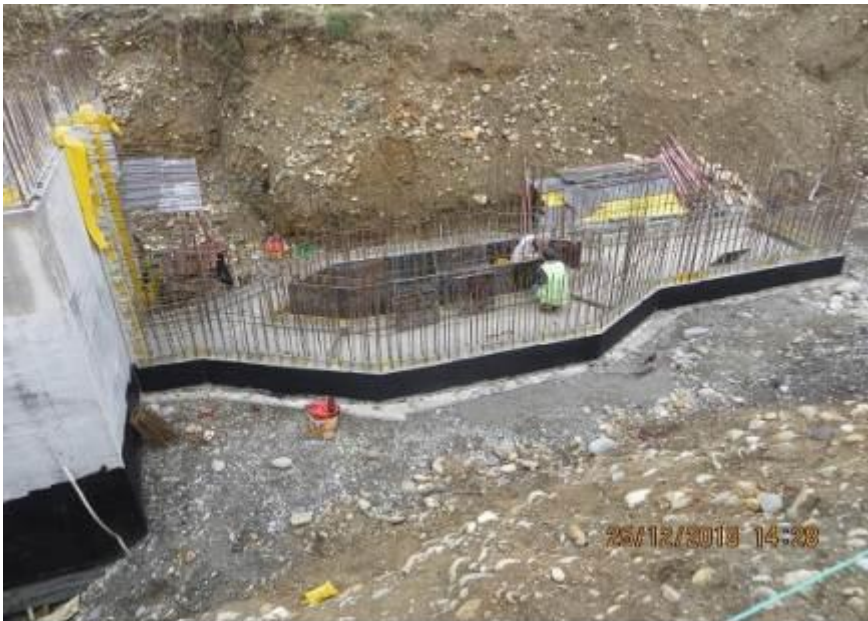
Photos of Reg-03/a project – Construction of Zugdidi WWTP
