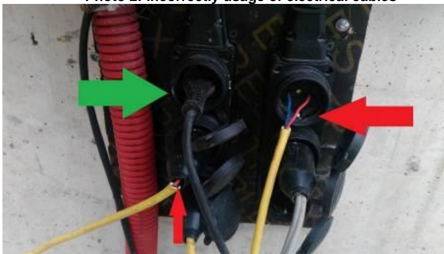
Photo 2: Incorrectly usage of electrical cables
