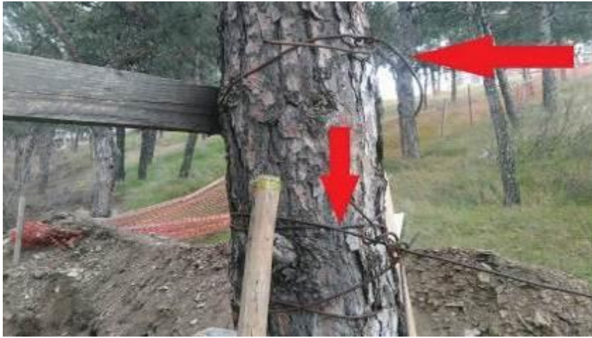
Photo 2: Incorrectly usage of electrical cables
