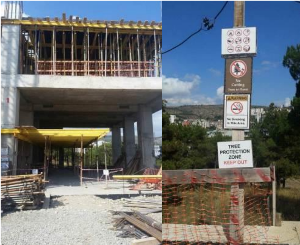
Photo: UWSCG Office Building, TBI-01
