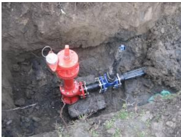
Kut-01: Network - Instalation of Hydrants:
