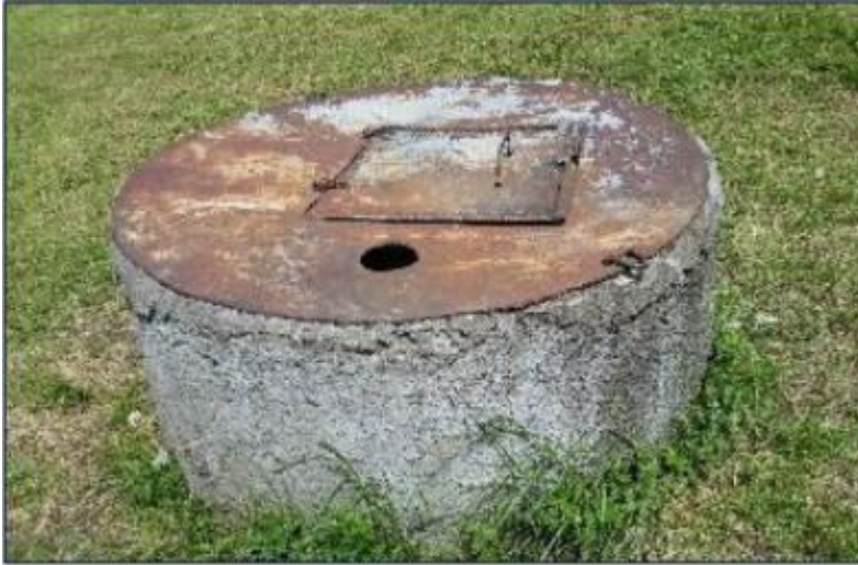
Chi-01: Perevisa existing reservoir
