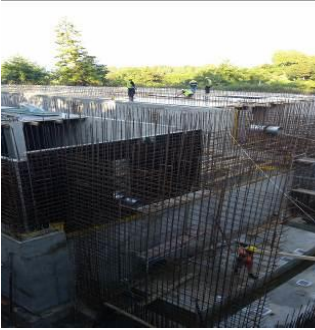
Ure-02: WWTP project site
