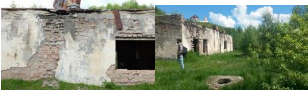
Figure 5: Old Wastewater Treatment Plant not in operation
