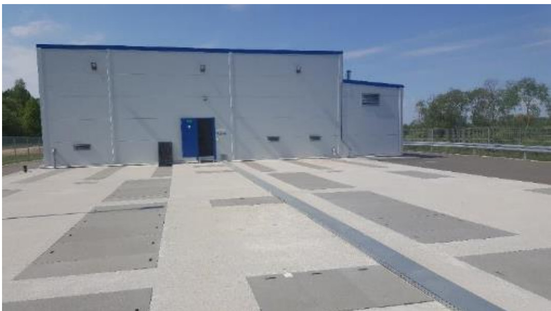
Figure 8: WWTP - Treatment system
