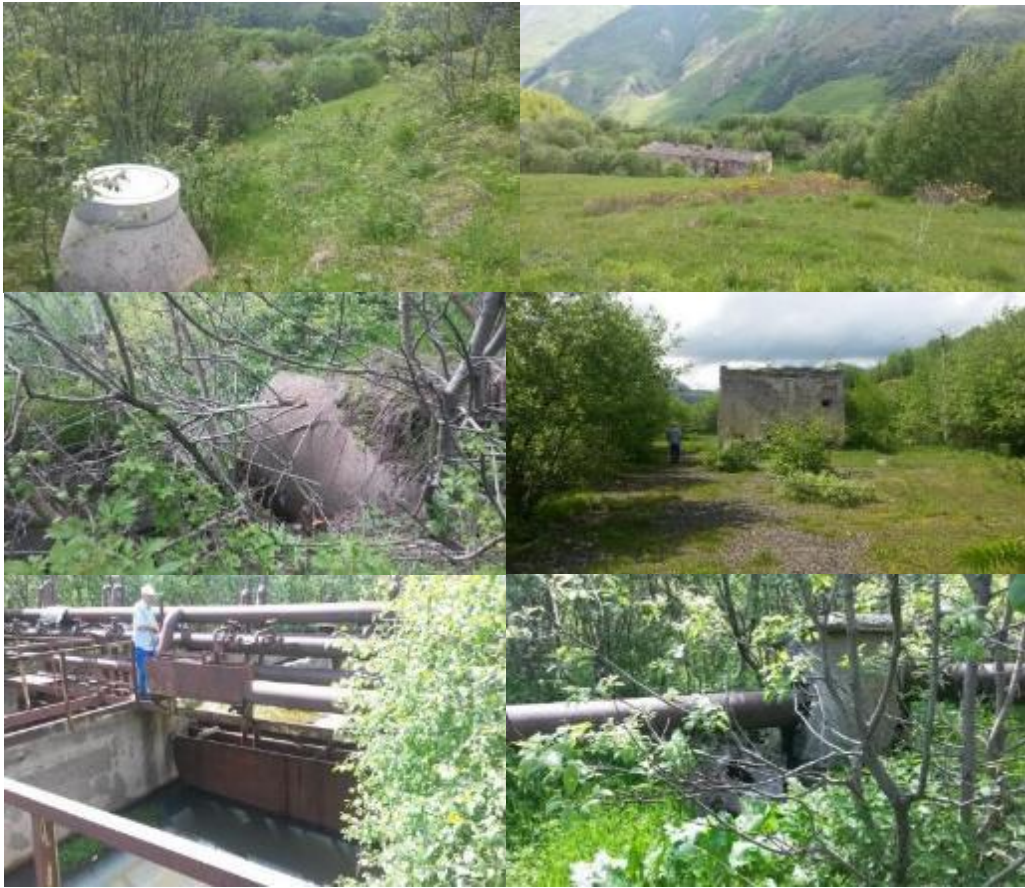
Figure 6: Alignment of the existing manholes and sewers (results of detailed survey)
