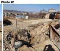
There is a dangerous of moving land on the upper perimeter of the reservoir, especially in rainy and windy weather, and to prevent this, protection must be taken immediately on the slope along the reservoir. Measures require an appropriate technical decision.
